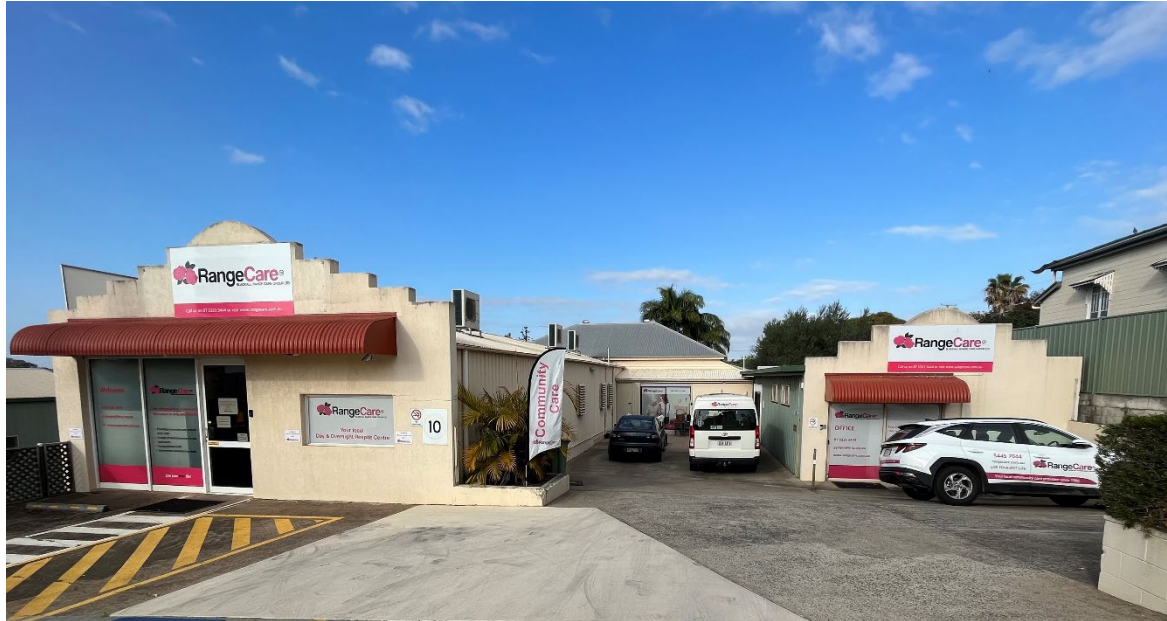
Gympie Day Respite Centre and Staff Offices on Barter St
